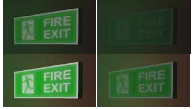
Figure 7: Illuminated exit signs (left column) are visible further than reflective exit signs (right column), which is achieved by adjustment of the transfer function.
